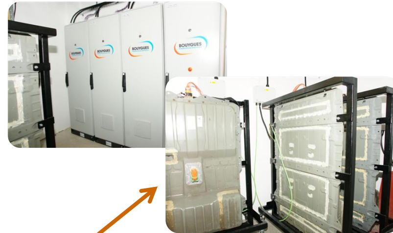
2 nd life EV battery ~16kWh
